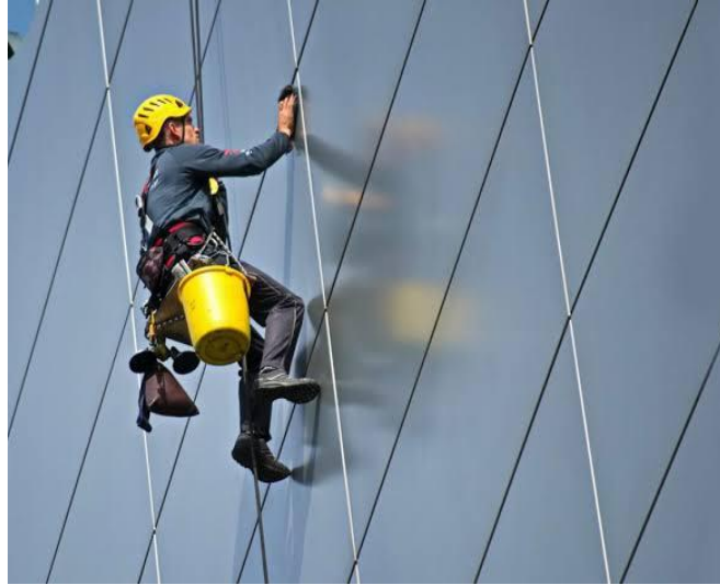
Gambar 2. 1 Metode Akses Tali rope access
